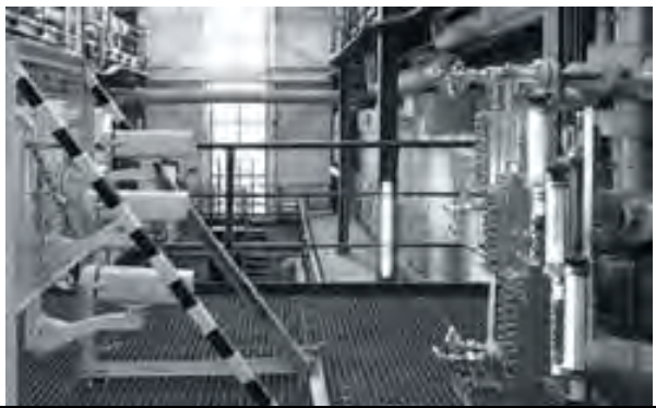
Illuminated boiler level gauges – any application to 200 bar
